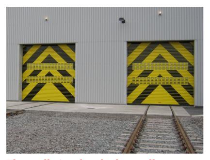
Thermally insulated robust roller shutters, manufactured and installed in accordance with BS EN 13241-1:2003 + A2:2016 & BS EN 12604:2017.
